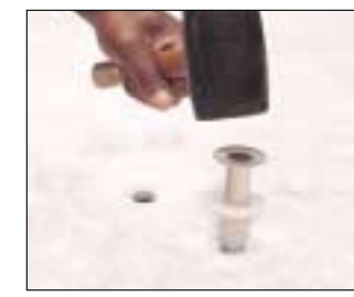
Step 2: Strike flange anchors with a rubber mallet
